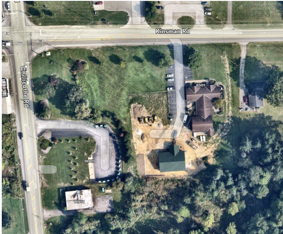
Russell Township Community Room
