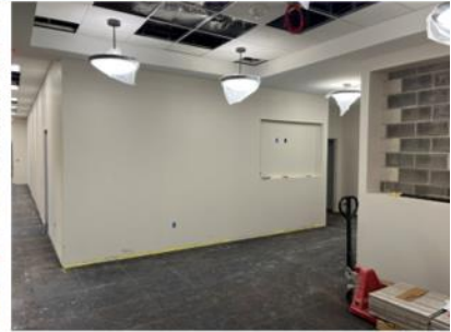
Entrance Lobby from Elevator
